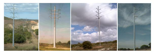
Figure 7.10: Examples of monopole distribution power line towers. Similar structures have been used for 400kV towers where space is limited
